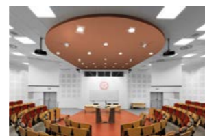
LIGHTING SCENE 1: During presentation the general lighting and the lighting of the presentation surface lights at 100%.
