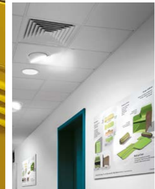
The school utilises the corridors often as a communication tool and places there information boards, message boards, pieces of work of its students or awards from various competitions. For highlighting these objects it is appropriate to use the accent lighting in the form of luminaires with a narrow luminous intensity curve or the wall-washers.
