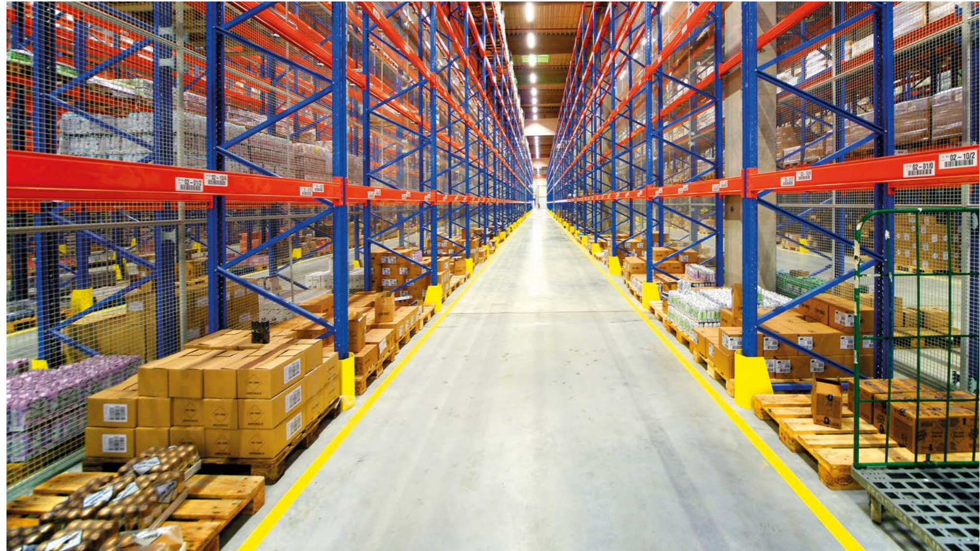
The presence detector switches on the luminaires in selected spaces when somebody is present and thus the lighting is really needed.
