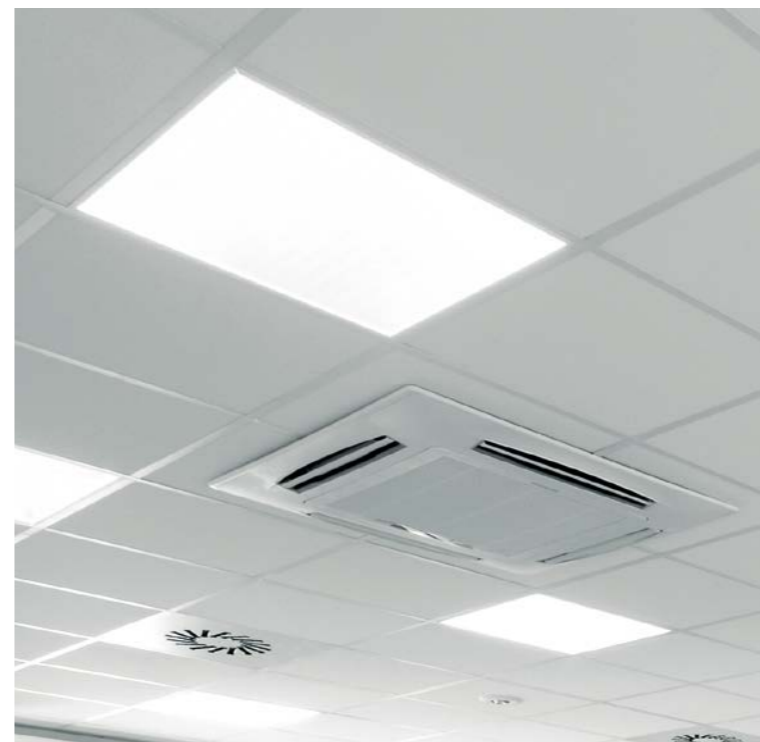
It is approximately valid that for 2.5 W of the luminaire energy 1 W of the air-conditioning energy is used, i.e. if the energy consumption of the lighting system increases, the energy consumption for the air-conditioning operation grows in direct proportion, too.
