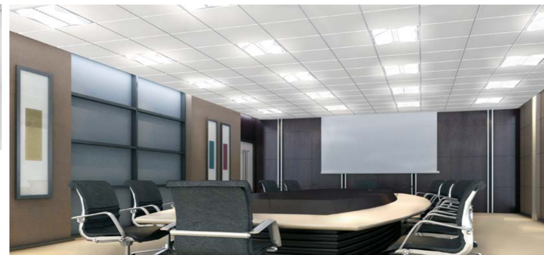
A similar result as with the suspension luminaires with direct and indirect characteristics of the luminous flux distribution can be achieved with recessed luminaires with a specially shaped diffuser.
