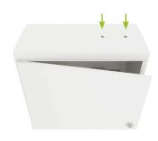
**1.** Using a drill create two holes in the casing of the streetlight cabinet.
